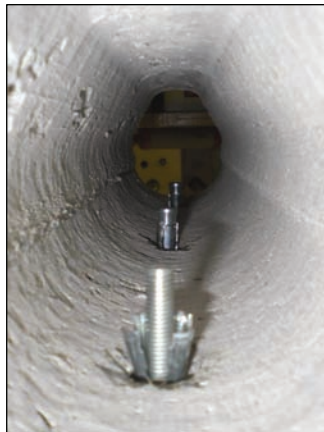
Figure 14: Flare-end anchors used in hollowcore concrete slab.
