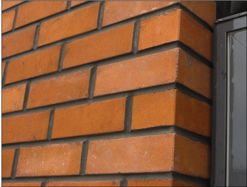
Figure 19: Solid blocks with dense structure, such as clay bricks, sand-lime bricks or natural stone.
