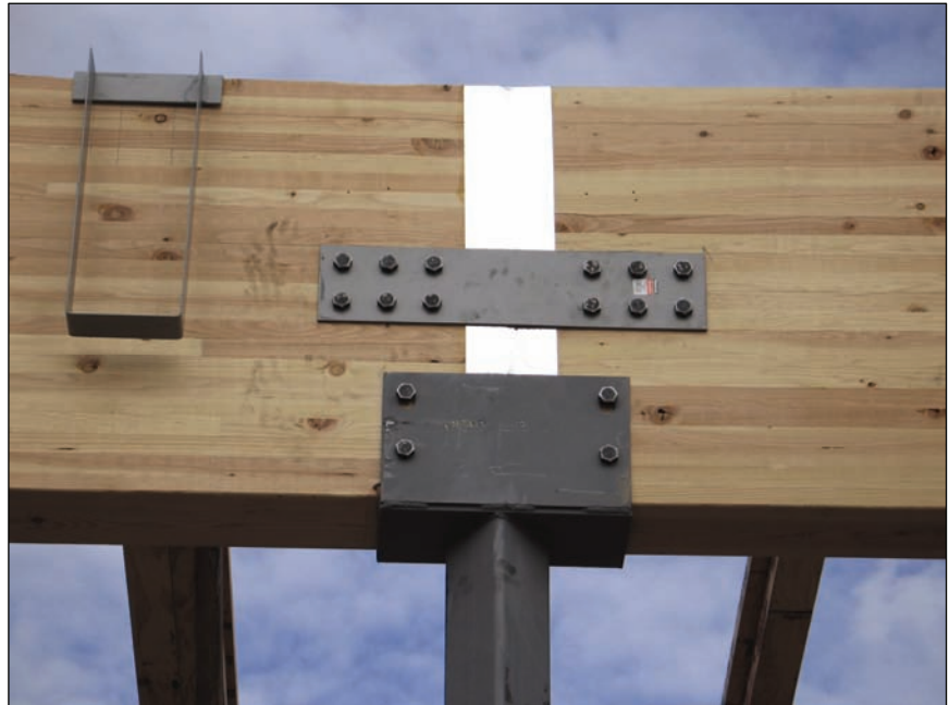
Figure 23: A glulam roof beam.
