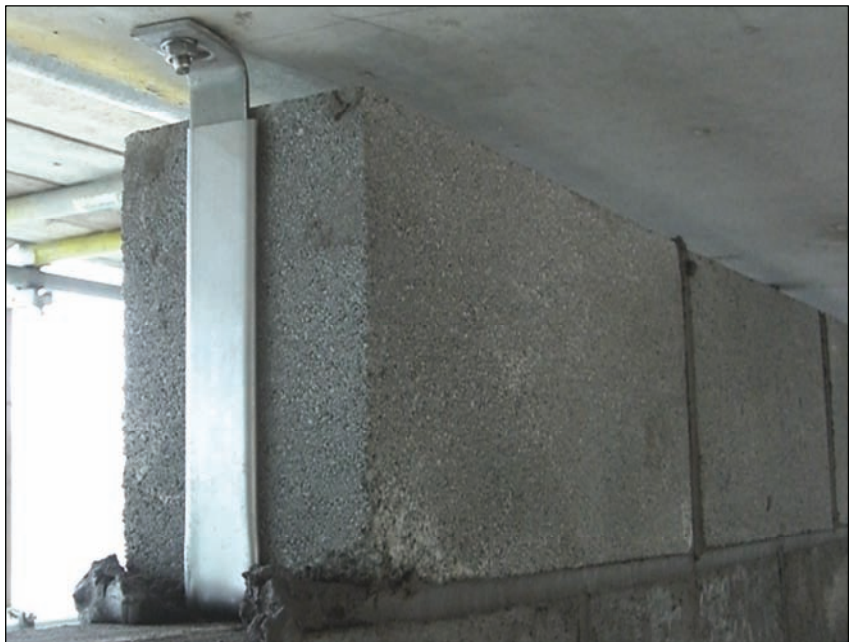
Figure 20: Solid blocks with porous structure, such as lightweight concrete blocks and Y-tong panels.
