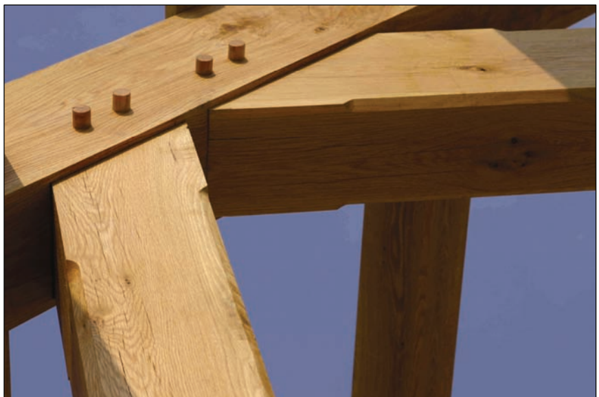
Figure 24: An oak frame for a building.
