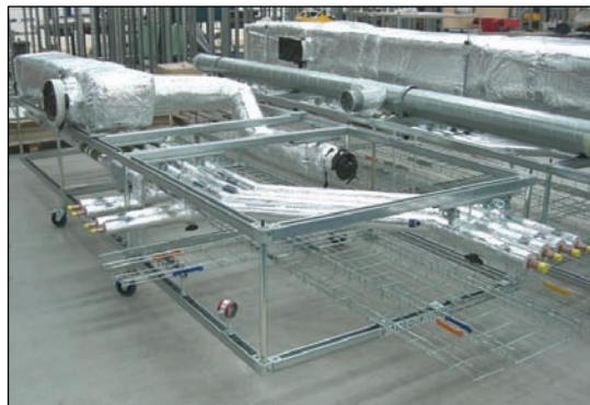
Figure 6: A prefabricated services module containing pipework, ductwork and electrical systems. This module will be elevated into position and fixed to the structure as a single element.
